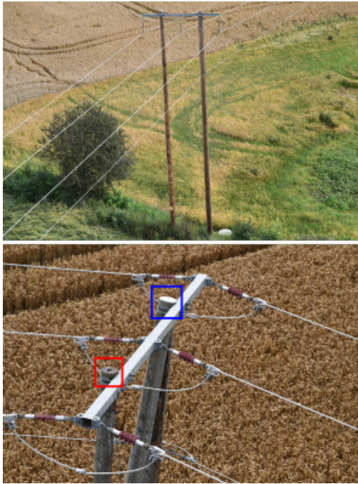
Fig. 3 Example of aerial helicopter images. On the bottom images, the bounding box of the "missing whole top cap" (red) and the "whole top cap" (blue) are visible.
